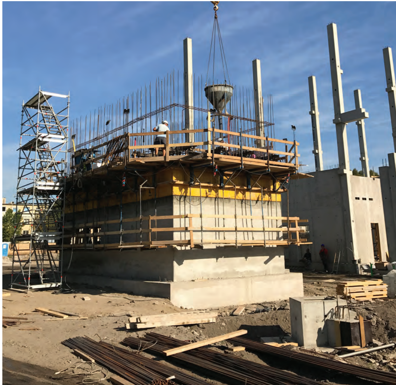
Structural construction of two stairwell shafts in Budapest. Year: 2017 Client: Moratus Ltd. Dimensions: Height: 16 m, each; Total surface area constructed by slipforming: 2,150 m 2
